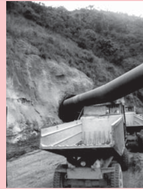
Building an Ethiopian hydroelectric power plant
