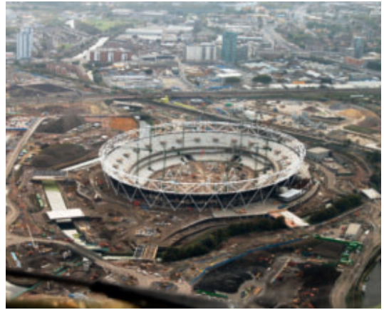
2 Construction at London 2012 Olympics site
