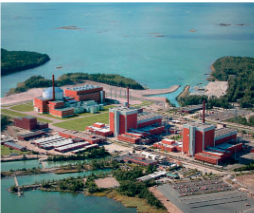
3 Olkiluoto nuclear power plant, Finland
