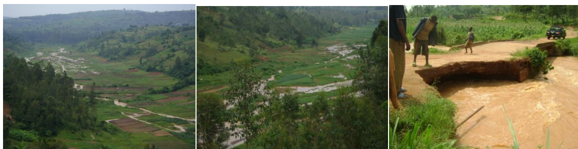
Figure 4.2: Crops flooded and bridge destroyed on 7 th Jan 2010, in Migina River which flows to Akanyaru River, Southern Rwanda
