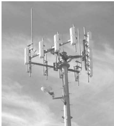
Figure 16.5 Sectorized base-station antenna.
