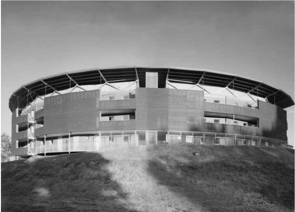
Figure 15.4 The CASPAR II apartment block, Leeds.
