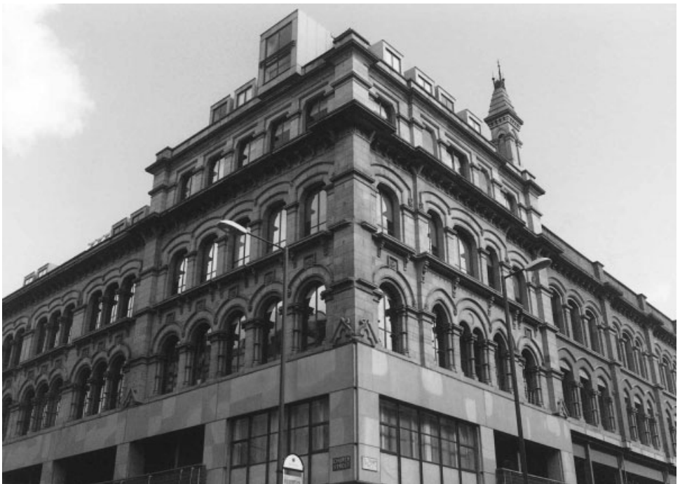
Figure 15.8 An external view of Smithfield Buildings, Manchester.
