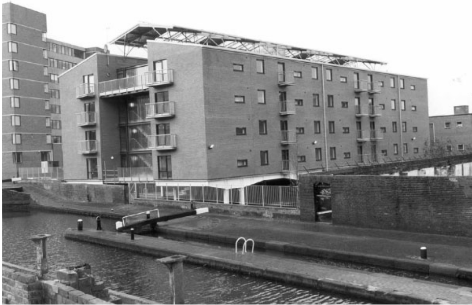
Figure 15.3 A view of the CASPAR I apartment block, Birmingham.
