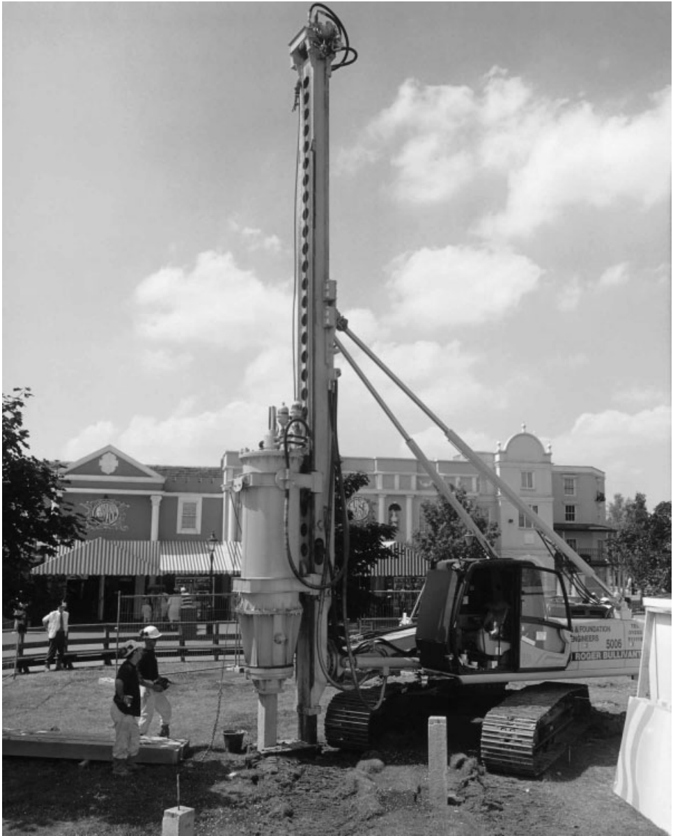
Fig. 7.3 Precast concrete driven piling rig.
