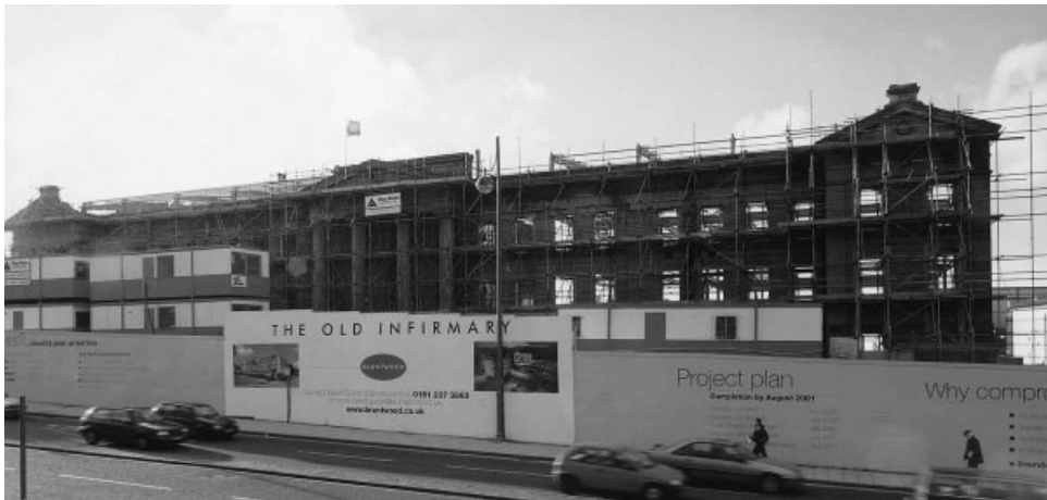
Figure 12.2 Good use of hoarding around a development site.
