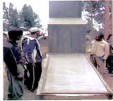
Figure 2b. Seed drying structure, front view
